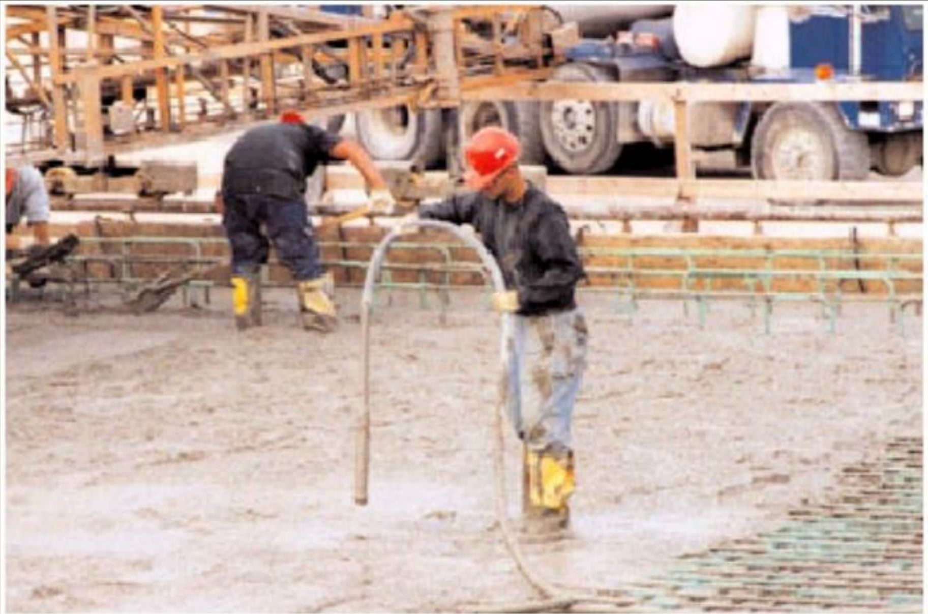
Fig. 11-11. Internal vibrators are commonly used to consolidate concrete in walls, columns, beams, and slabs. (69970)
