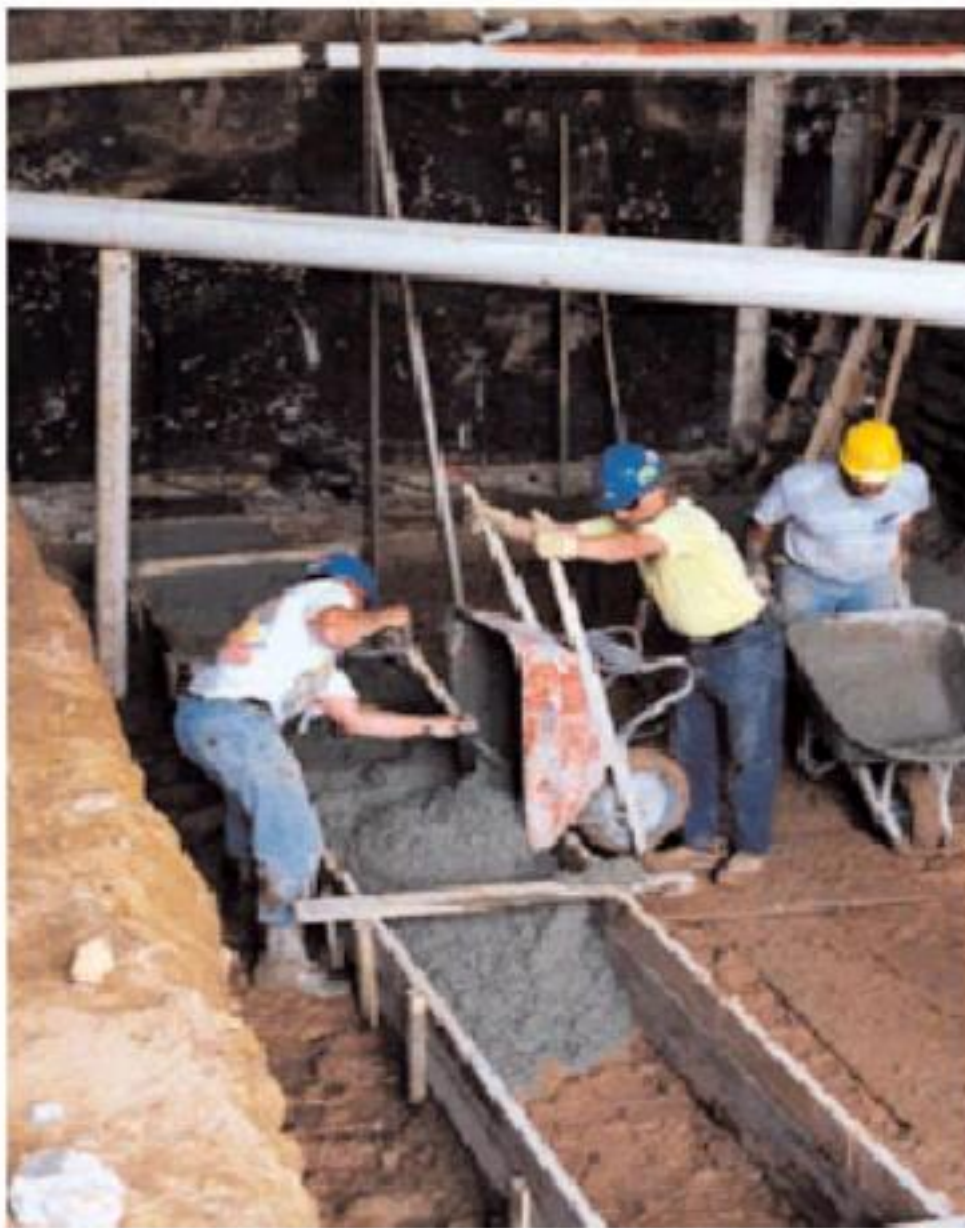
Fig. 11-4. Wheelbarrows are used to place concrete in areas that are not easily accessed by other placement methods. (69929)
