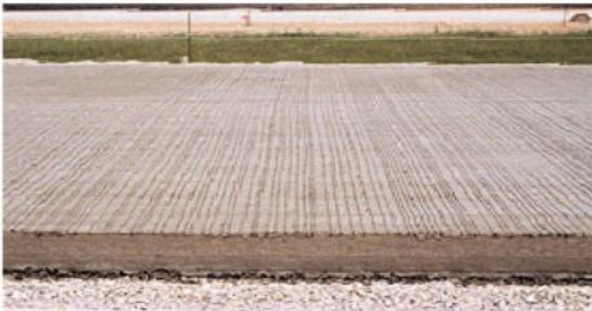
Fig. 11-21. (top) This machine is tining the surface of fresh concrete. (bottom) Tining of pavements improves tire traction and reduces the risk of hydroplaning. (69944, 69945)
