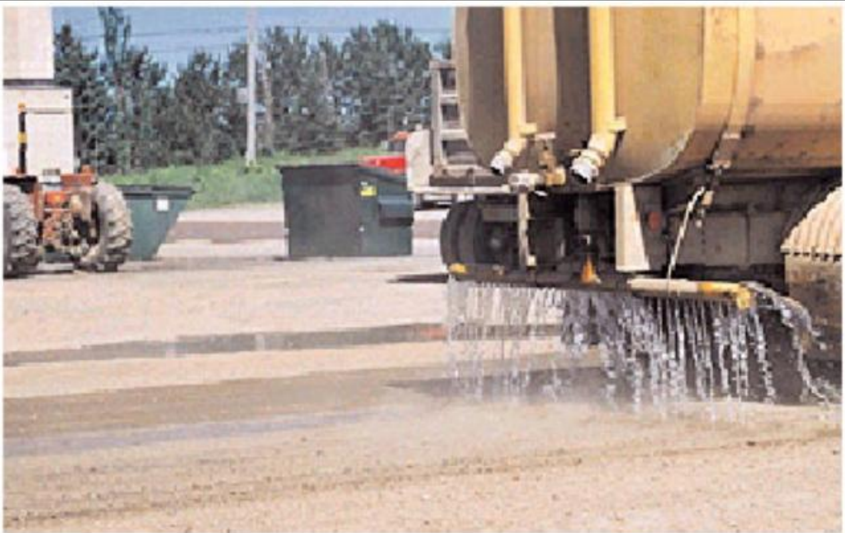
Fig. 11-2. Water trucks with spray-bars are used to moisten subgrades and base course layers to achieve adequate compaction and to reduce the amount of water drawn out of concrete as it's placed. (69931)
