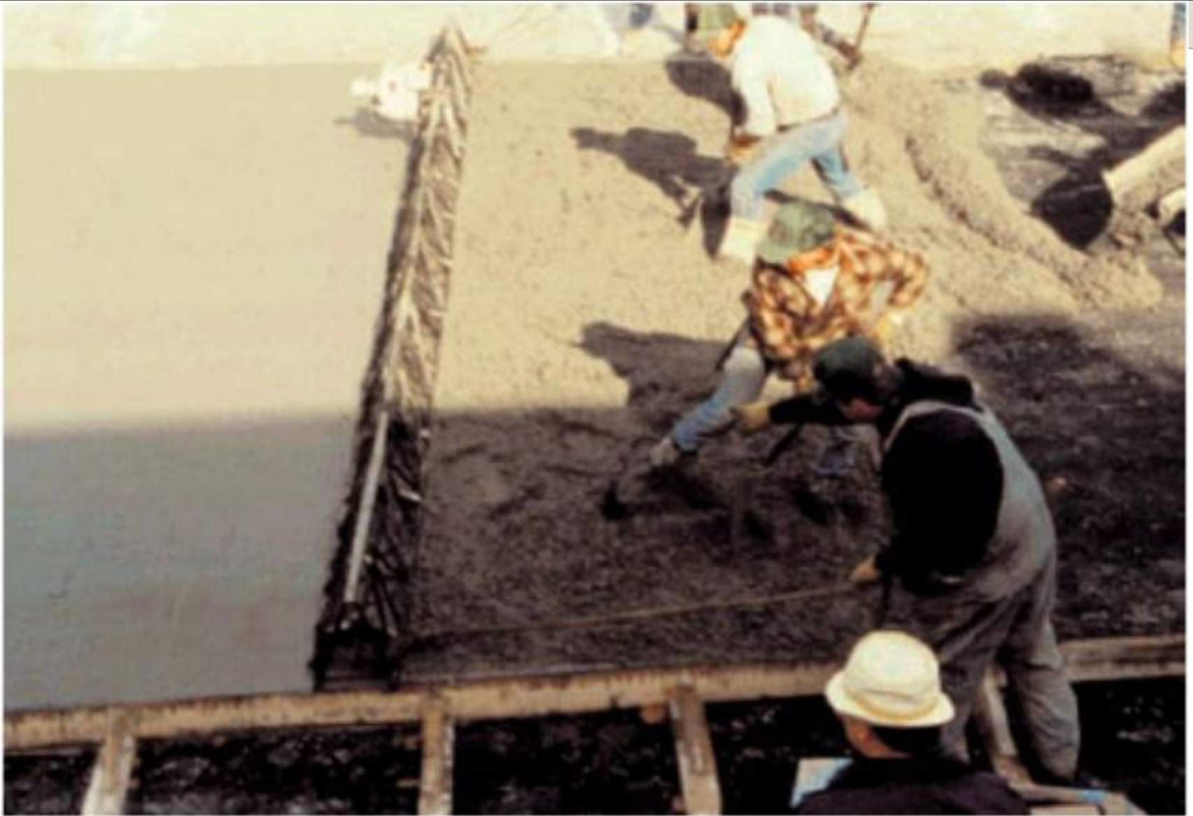
Fig. 11-12. Vibratory screeds such as this truss-type unit reduce the work of strikeoff while consolidating the concrete. (55801)
