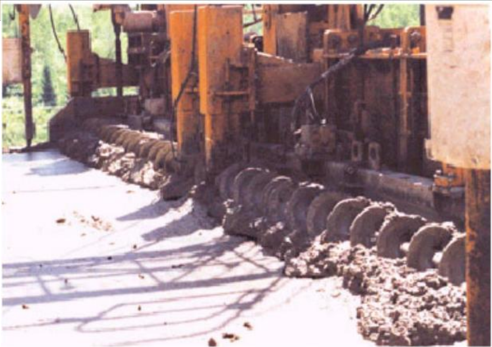
Fig. 10-16. The screw spreader quickly spreads concrete over a wide area to a uniform depth. Screw spreaders are used primarily in pavement construction. (69895)
