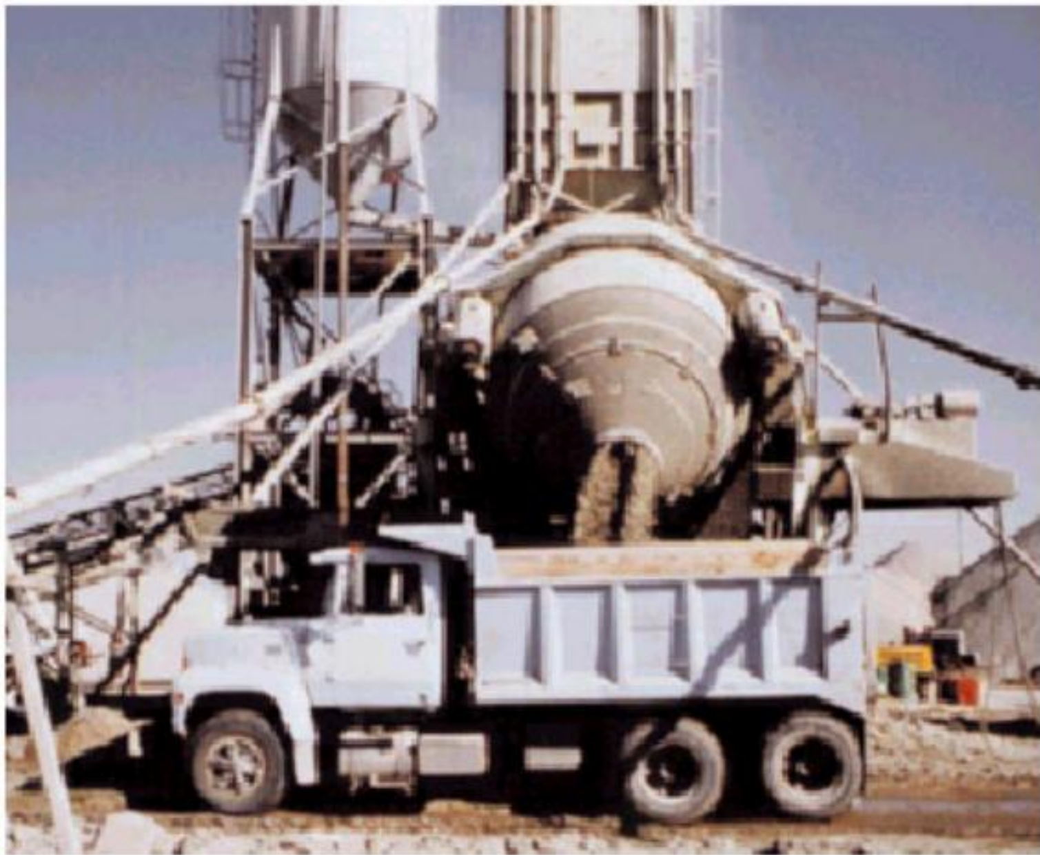
Fig. 10-2. Concrete can be mixed at the jobsite in a stationary mixer. (58642)
