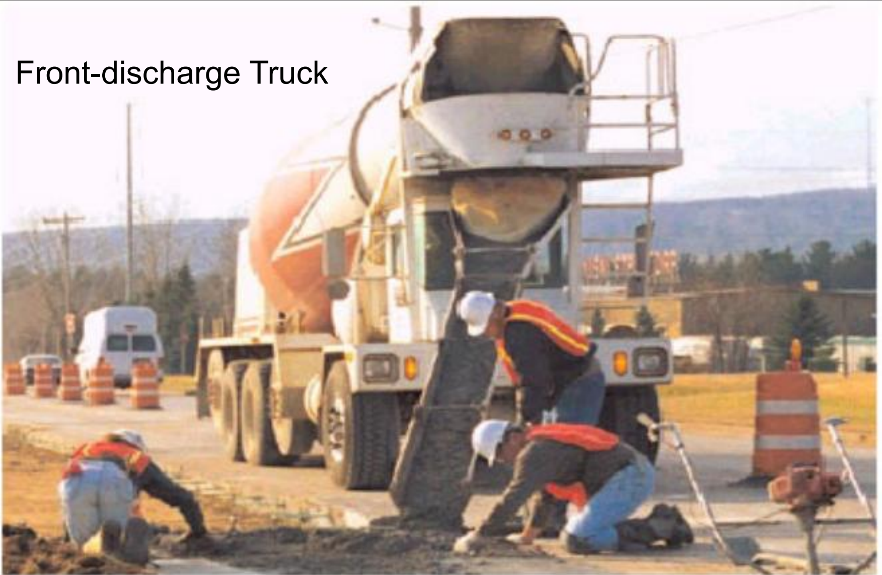
Fig. 10-10. In comparison to conventional rear-discharge trucks, front-discharge truck mixers provide the driver with more mobility and control for direct discharge into place. (70006)
