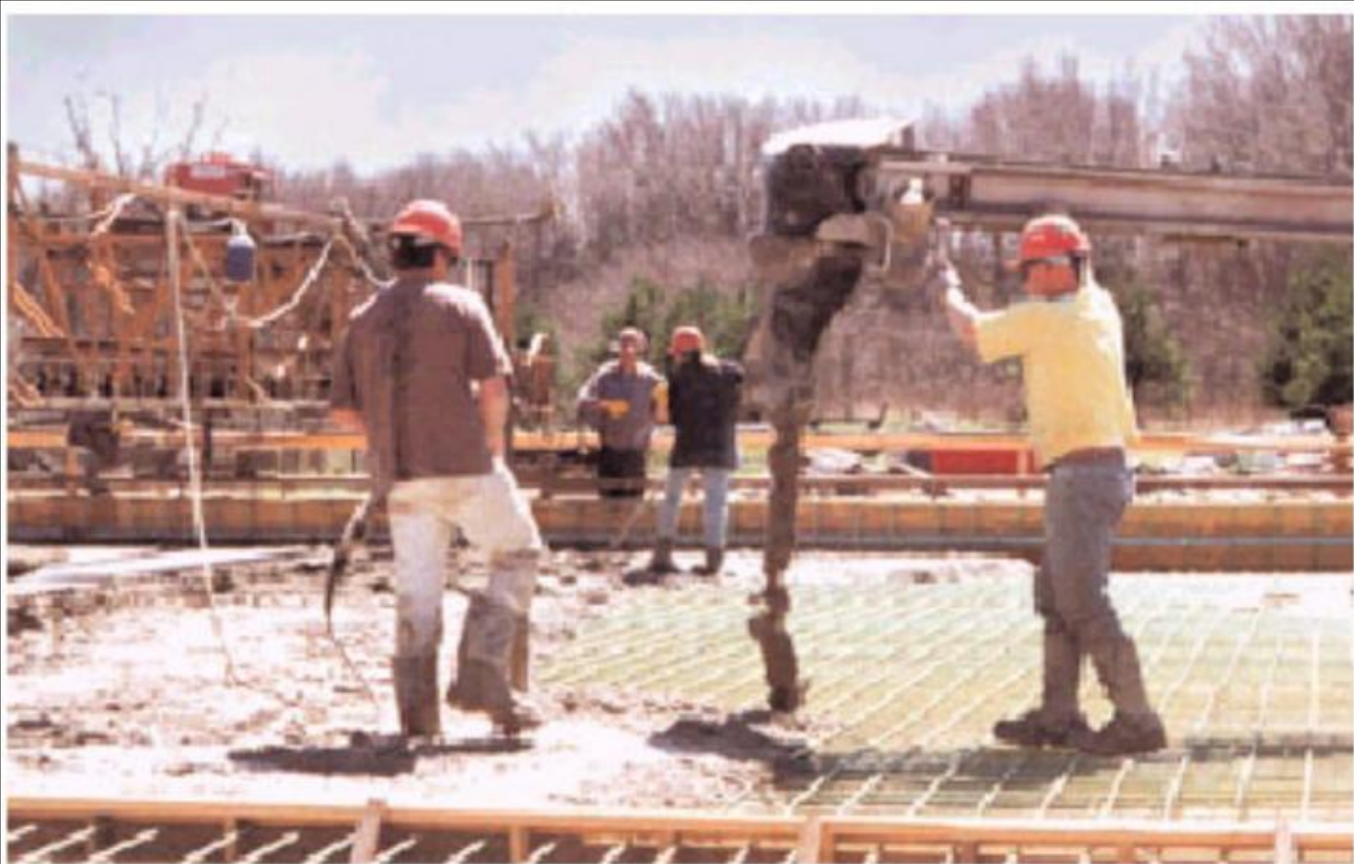
Fig. 11-5. The swing arm on a conveyor belt allows fresh concrete to be placed fairly evenly across a deck. (70002)
