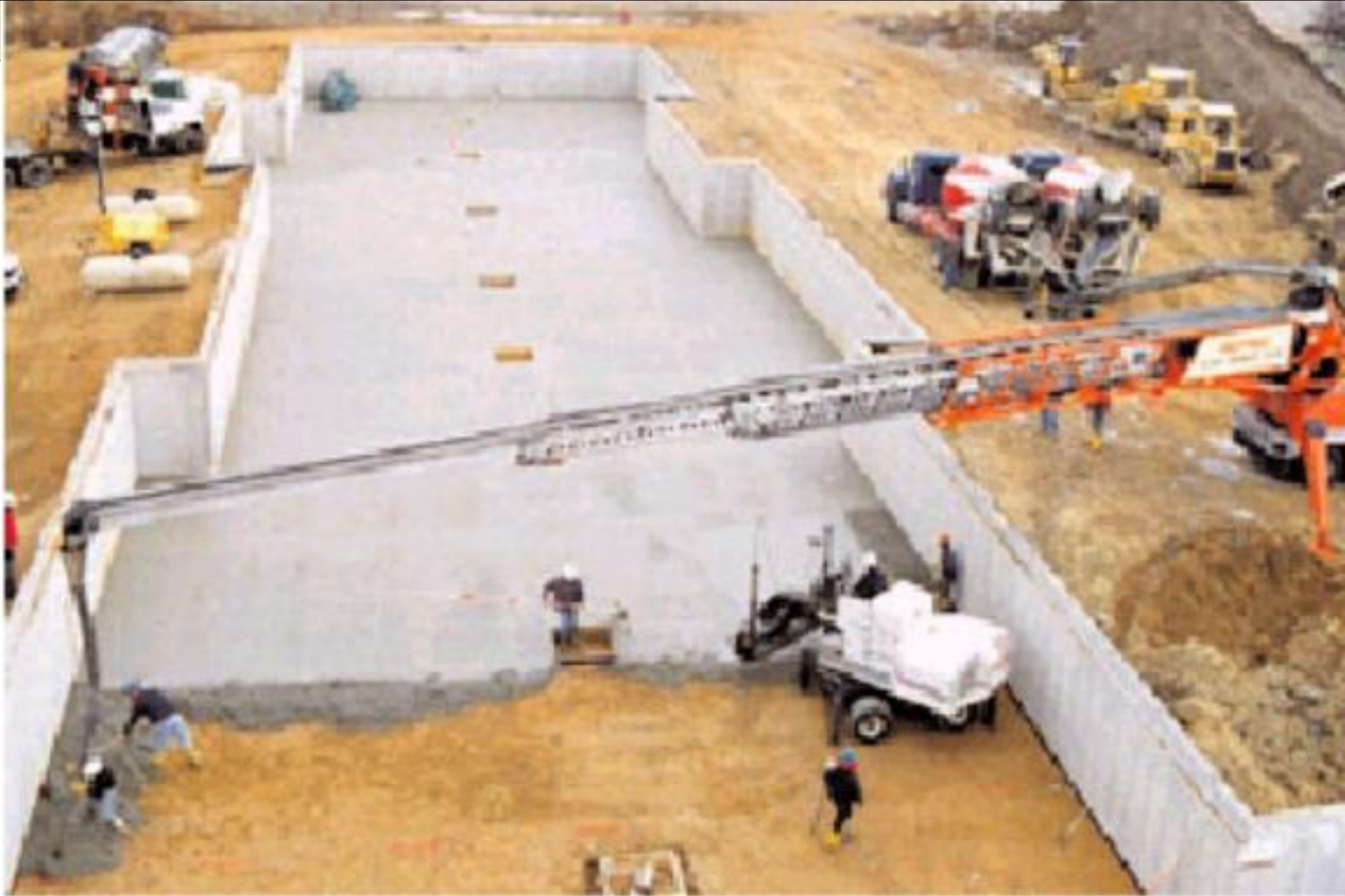
Fig. 10-13. The conveyor belt is an efficient, portable method of handling concrete. A dropchute prevents concrete from segregating as it leaves the belt; a scraper prevents loss of mortar. Conveyor belts can be operated in series and on extendable booms of hydraulic cranes. (69896)
