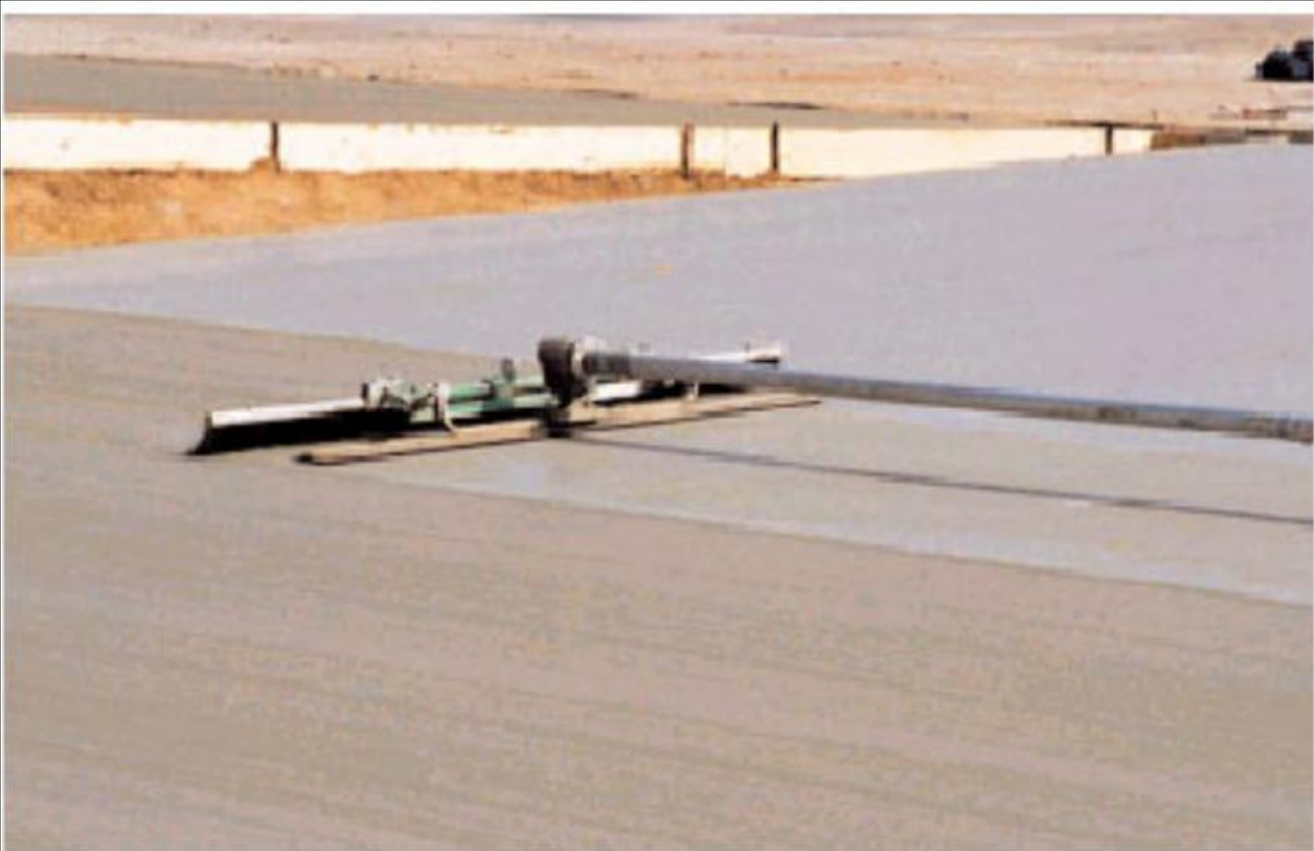
Fig. 11-20. Brooming provides a slip-resistant surface mainly used on exterior concrete. (69943)
