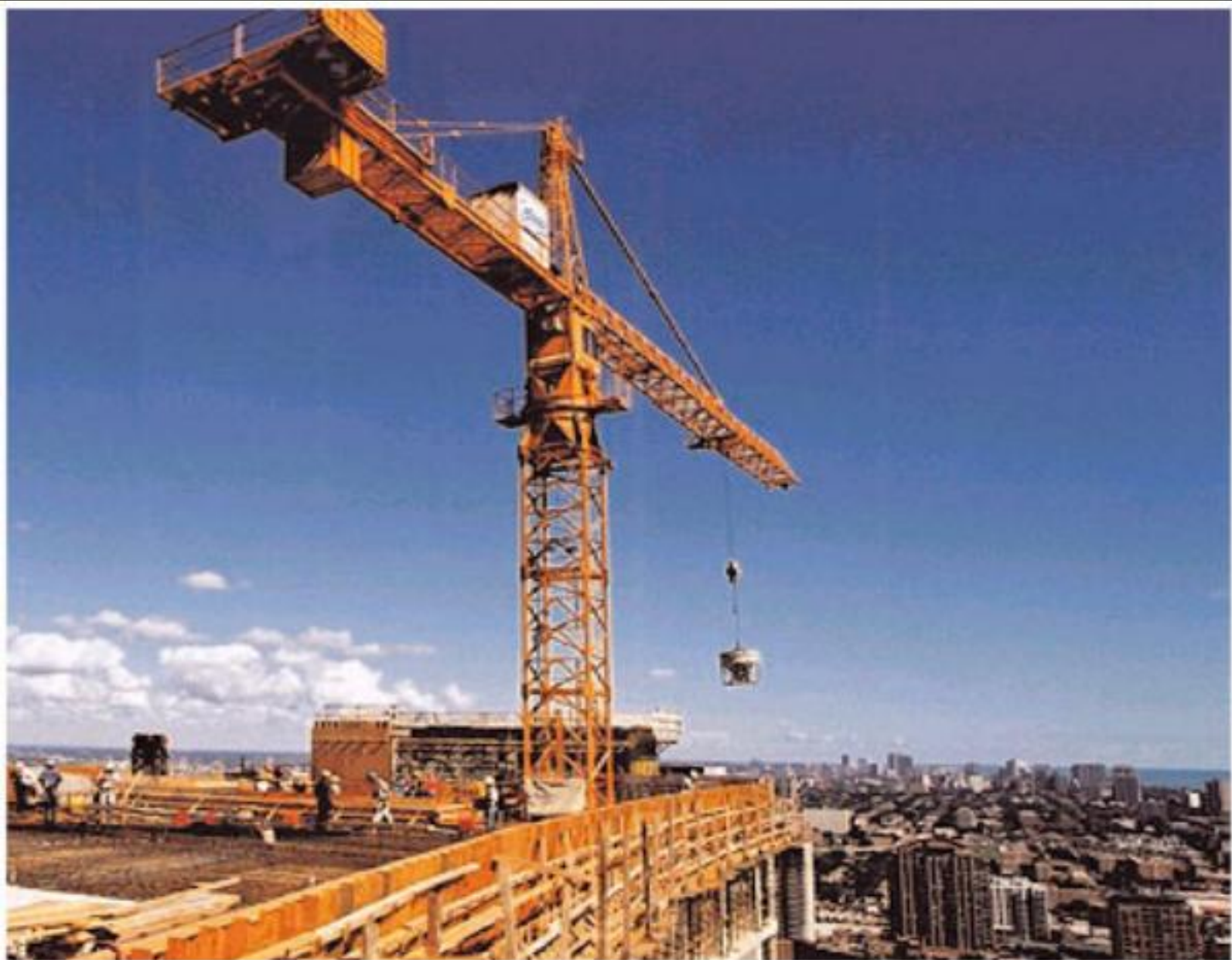
Fig. 10-12. The tower crane and bucket can easily handle concrete for tall-building construction. (69969)
