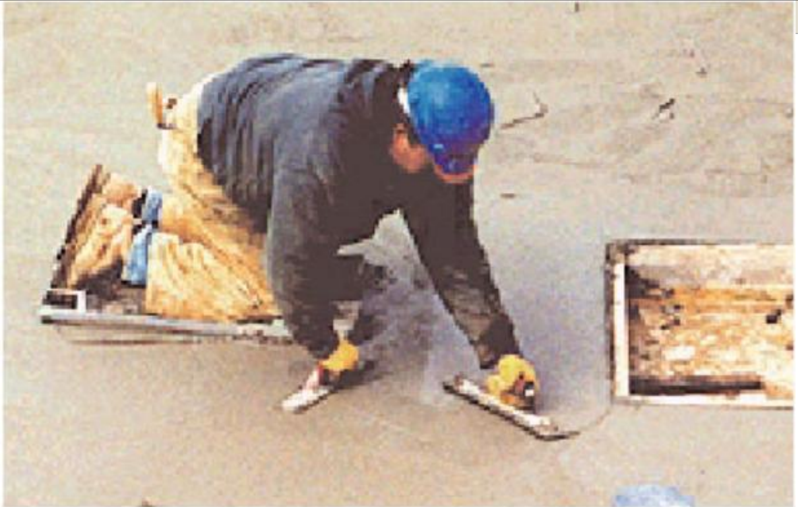
Fig. 11-19. Hand floating (right hand) the surface with a hand float held flat on the concrete surface and moved in a sweeping arc with a slight sawing motion. Troweling (left hand) with blade tilted is performed before moving the knee-boards. (69933)
