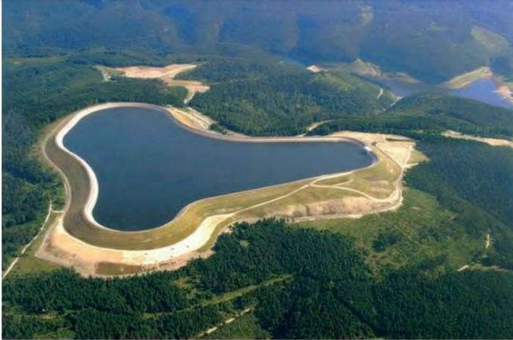
Pumped Hydro Storage
