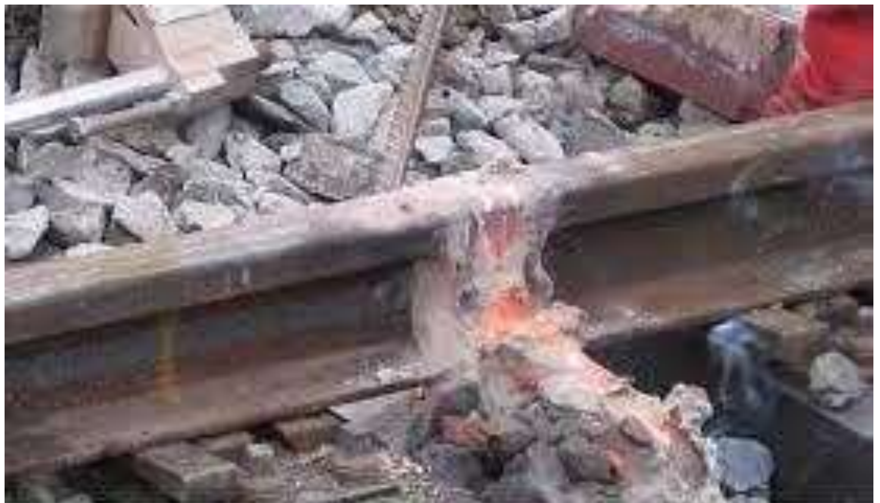
Thermit Welding on Railway Track
