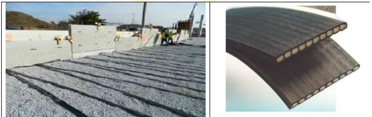
Fig.1: Geo-strip Reinforcement
