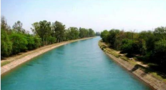
Fig 4: Sirhind Feeder Canal, India
